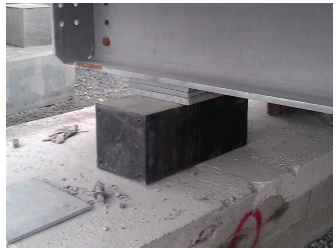
STRUXURE 10" x 10" x 20" storage support for 90,000 lb. bridge panel
